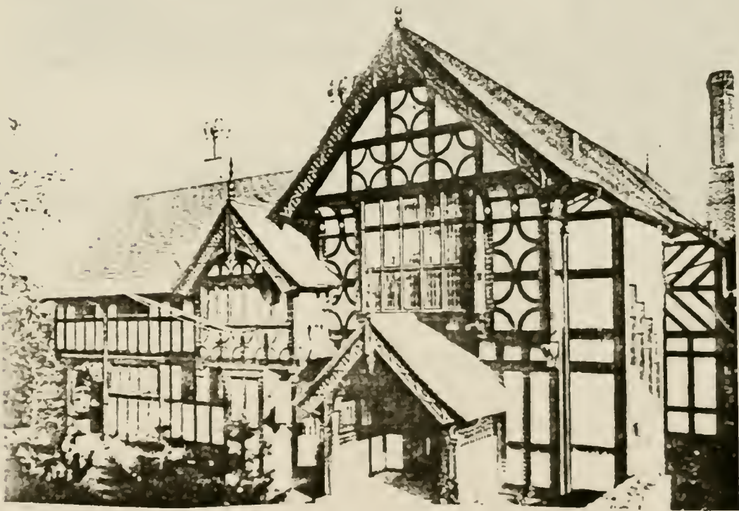
4 The Front Facade of the Sharpe Residence.
